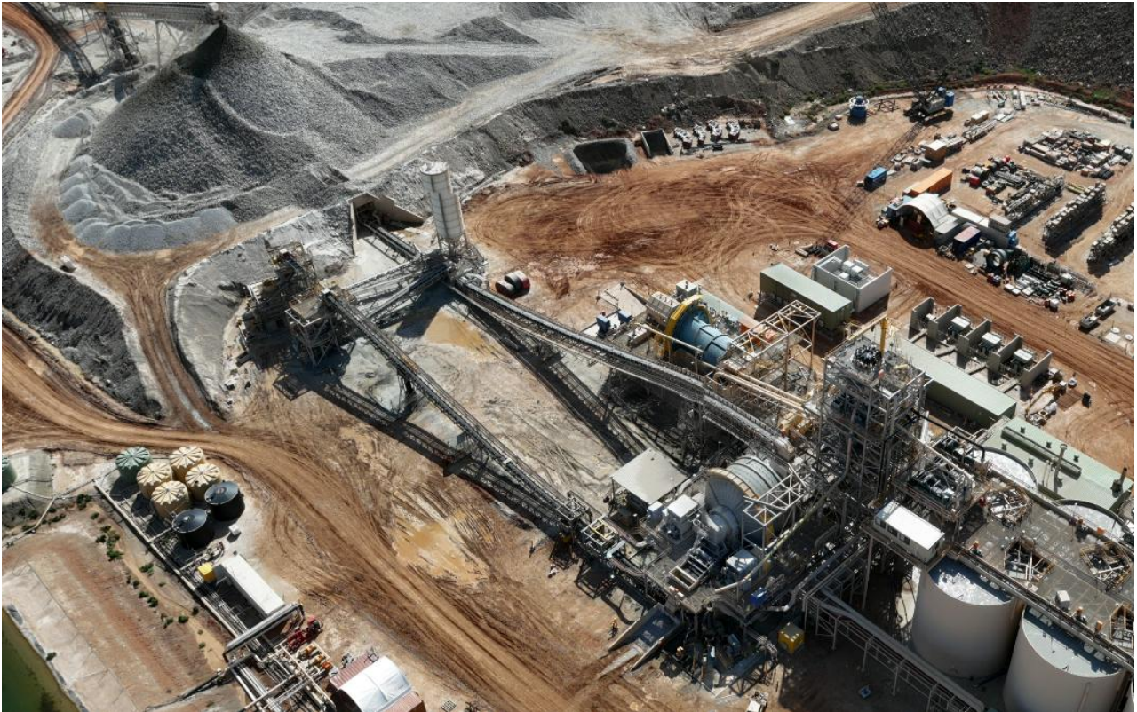
Figure 4: Aerial view highlighting new ball mill and pebble crusher
