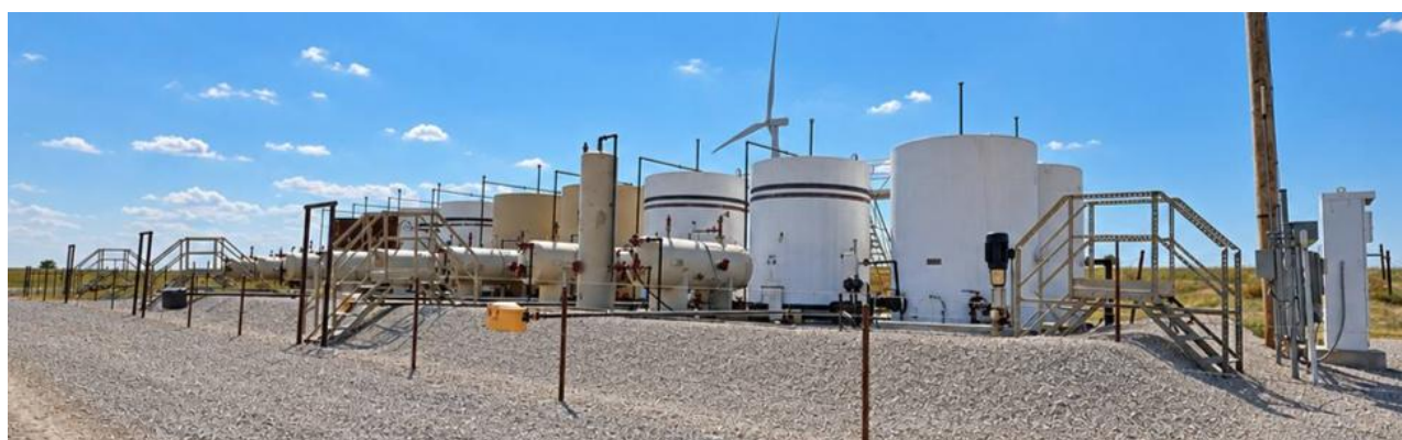
Figure 1,2,3 Photos Taken by Management during field inspection of acquisition properties in Oklahoma
