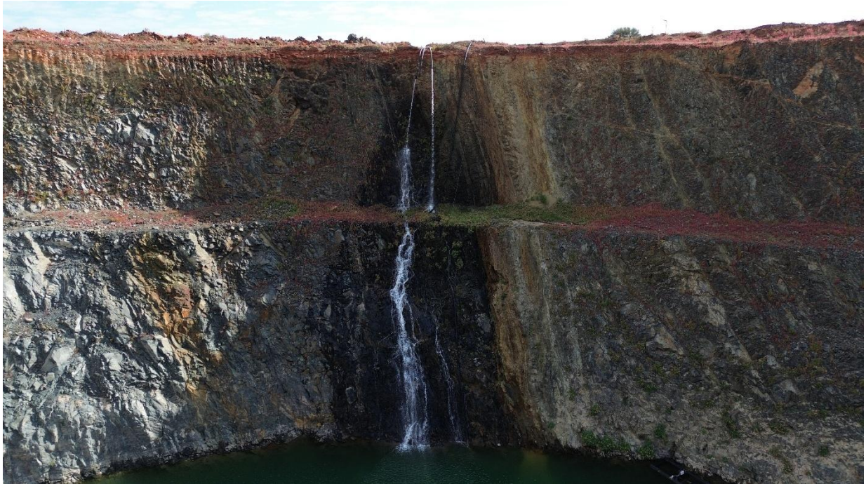
Figure 3: Water discharging into the Eclipse Pit from the Comet underground dewatering operation.
