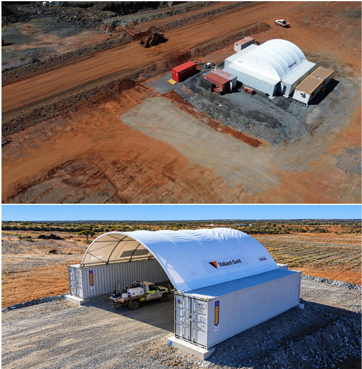
Figure 4: Workshop, office and medical facilities installed at Comet.
