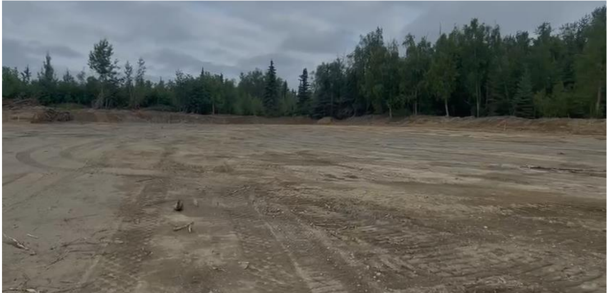
Figure 2. Port MacKenzie antimony processing plant site early earthworks
