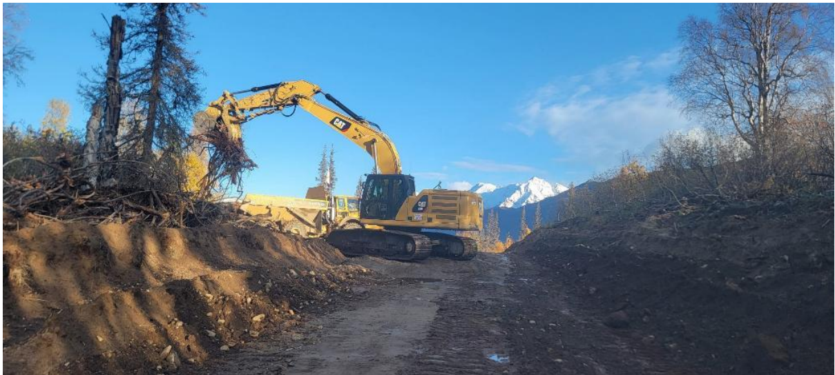
Figure 3. Korbelt-Stibium access road construction works
