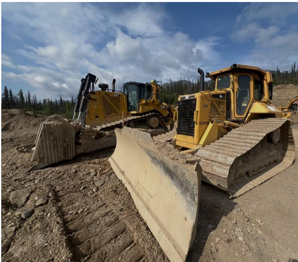
Figure 4. Whiskey Bravo airstrip expansion construction works
