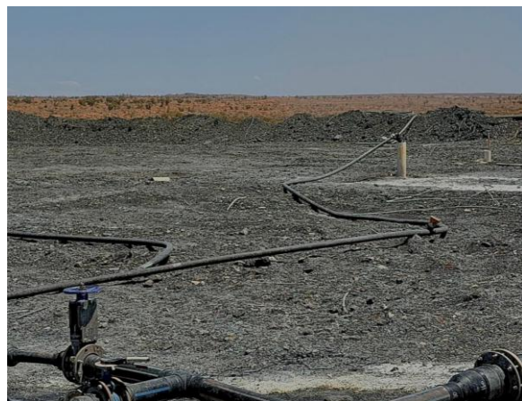
Figure 6: Low pressure solution application
