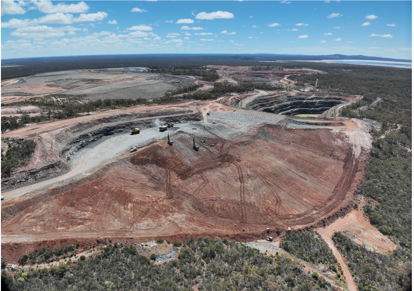
Mining underway at Green Lantern Stage 2
