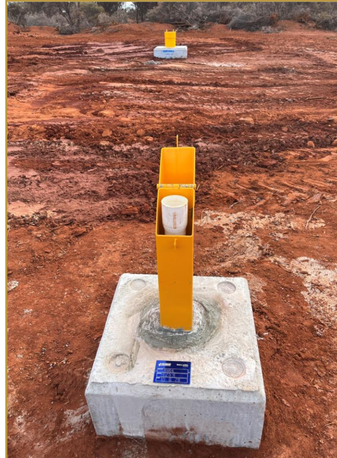
Production bore background and monitoring bore foreground
