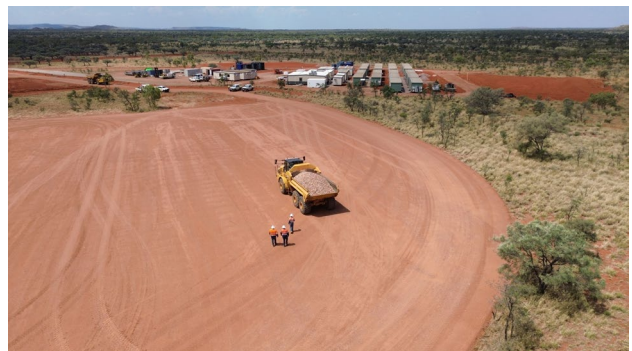
Village civil works under construction
