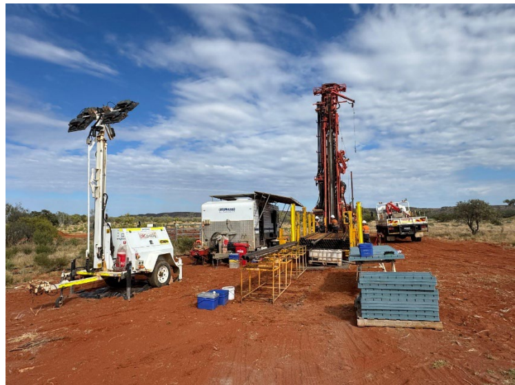
Drilling at Jervois Site
