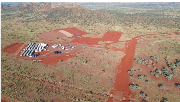
Construction village installed – civil works underway for the village and access roads.
