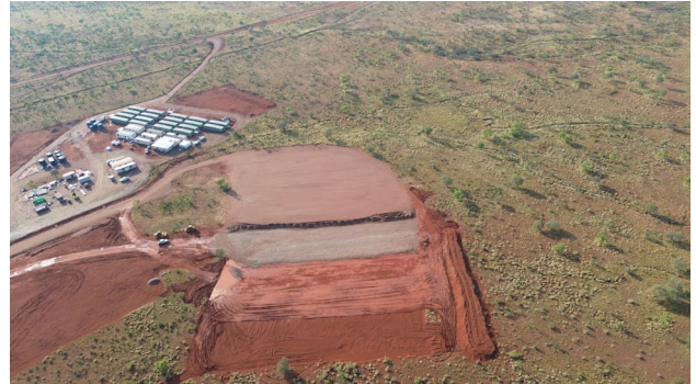
72 room construction camp installed and 180 room village under construction
