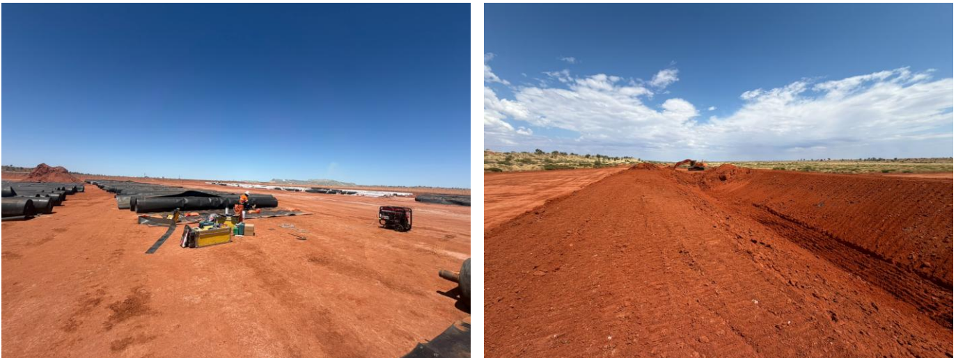
Figure 2: Evaporation pond 4 works (LHS) and blind bore pad construction (RHS).
