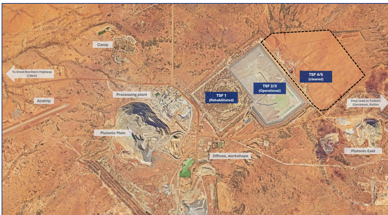
Figure 3: Aerial image of Plutonic site, showing existing TSF cells and cleared area for construction of TSF 4/5
