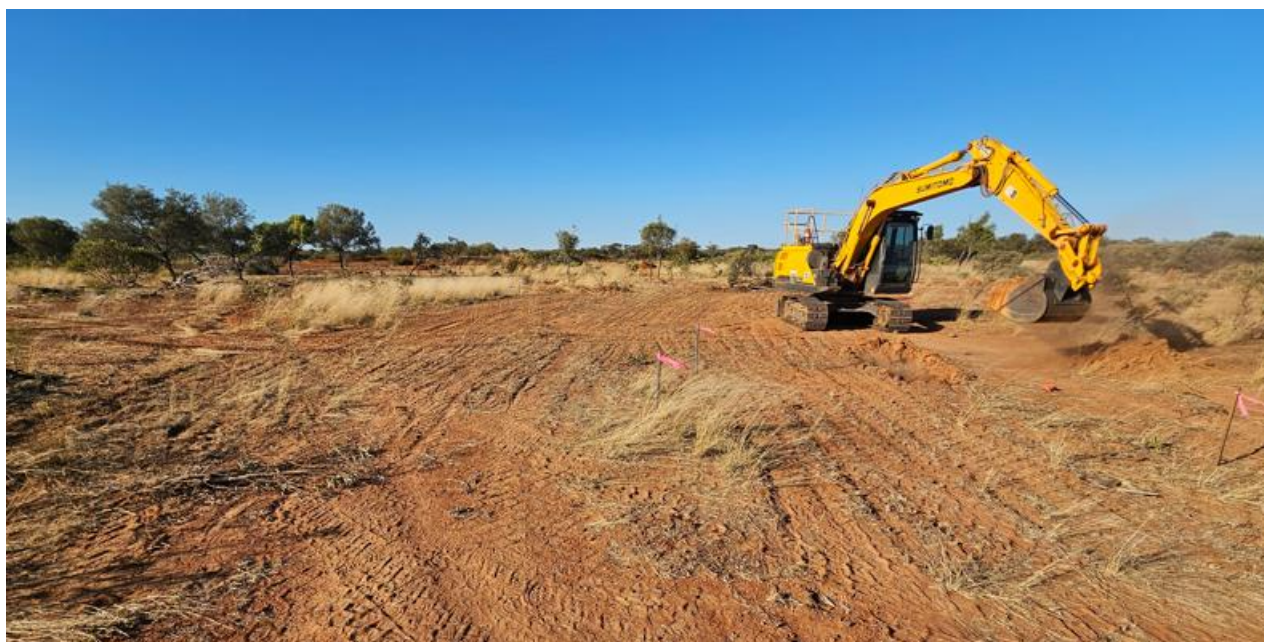
Figure 1 – Earthworks and drill pad preparation at Orlando.
